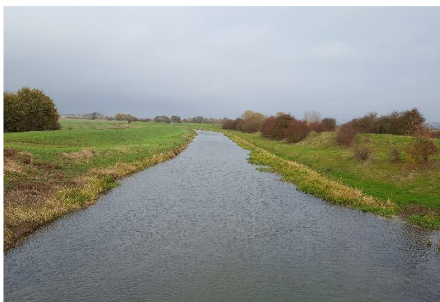
Photo 1 - River Witham looking downstream
