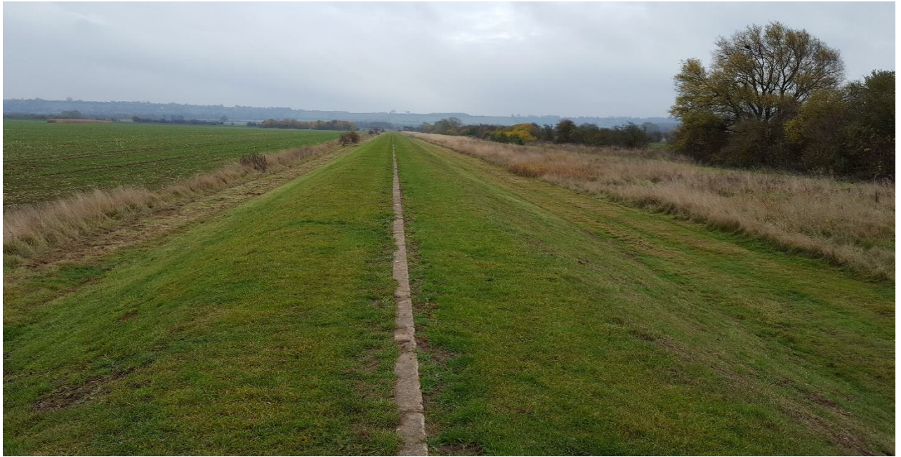
Photo 6 - Lincoln Washlands FAS embankment
