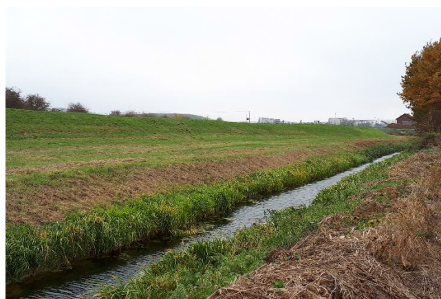
Photo 2 - Hykeham Pump Drain South looking south towards Lincoln Washlands FAS
