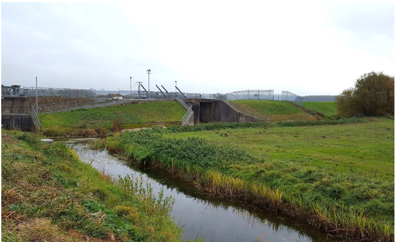
Photo 5 - Lincoln Washlands FAS inlet/outlet sluice
