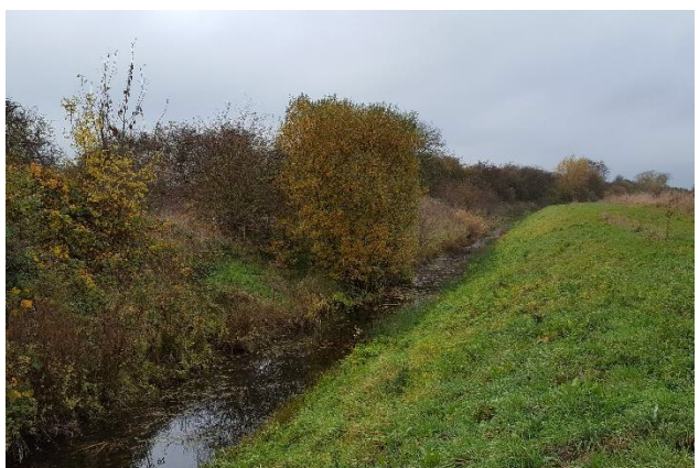
Photo 3 - Washland Soke Dyke looking west
