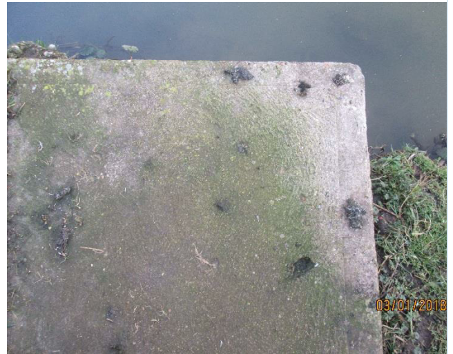
Photo 18: Otter spraint on concrete platform at TN8 next to River Witham
