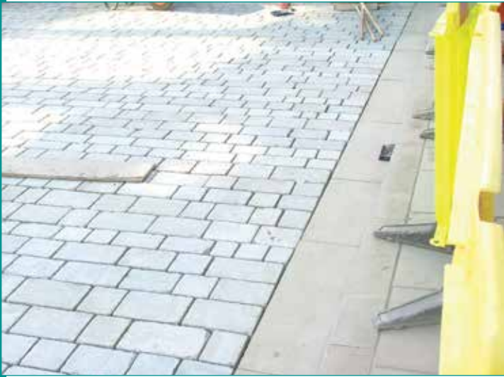
Danesgate surfacing under construction
