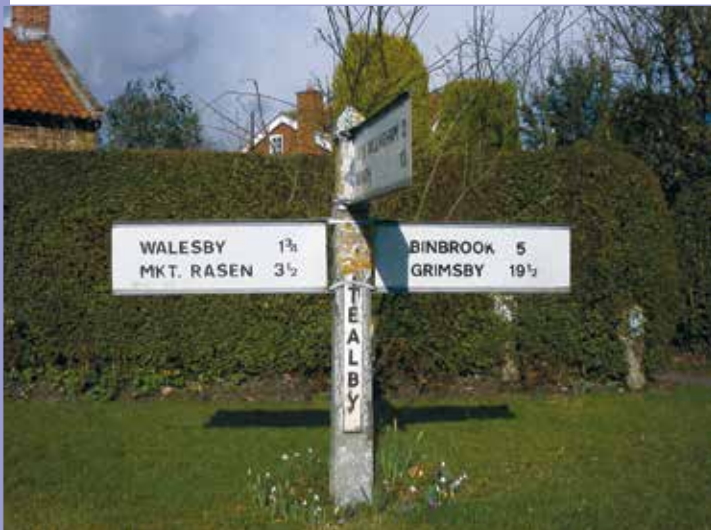
Concrete posts with wooden arms, like this example in Tealby, are more prevalent in the north of the county. Note the replacement of the modern reflective metal directional arms with wooden arms.
