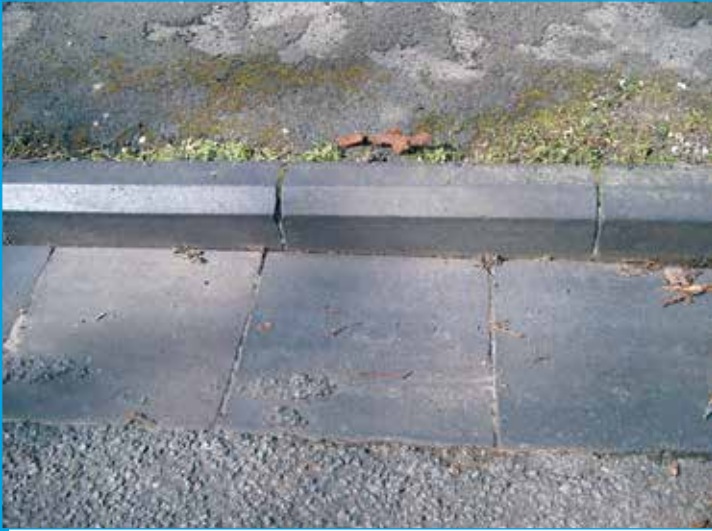
Historic blue brick kerbing and drainage, Woodhall Spa, in a Conservation Area. These should be retained wherever possible, and where replacements are necessary, these should be sympathetic. Care should be taken when resurfacing the road that this type of feature is not damaged or covered up.
