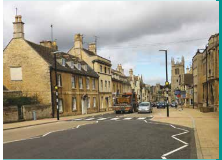
The scheme following completion
