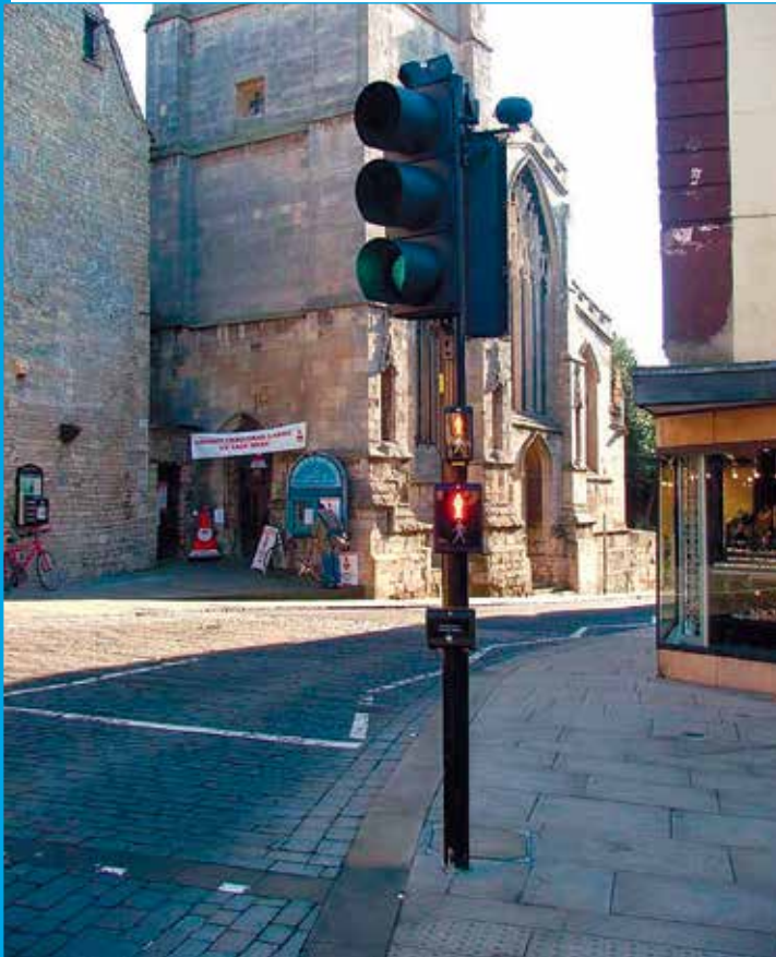
Reflective white edging has been omitted from the design of these signal heads in Red Lion Square, Stamford.
