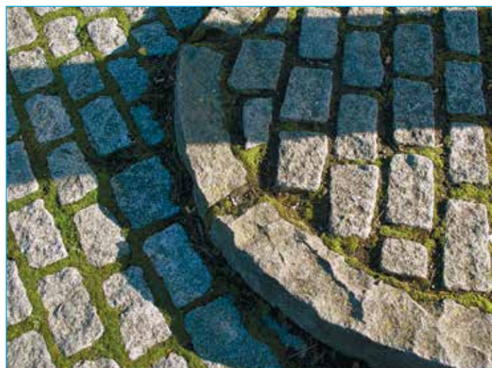
Granite setts and kerbing have been used in a recent scheme in the centre of Binbrook, which is also a Conservation Area, and in the Lincolnshire wolds AONB. (See section 4.3.6 Materials).
