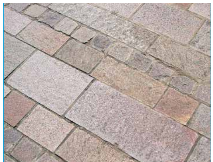
■ Porphyry (granite) paving in Coningsby town centre; attractive laying pattern using a combination of sizes.
