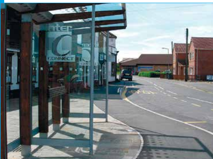
■ Porphyry (granite) paving in Coningsby town centre; attractive laying pattern using a combination of sizes.
