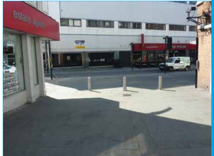
Wide controlled crossing across Silver Street, in Lincoln's Cultural Quarter. This measure is intended to improve pedestrian links between the northern and southern parts of the city.
