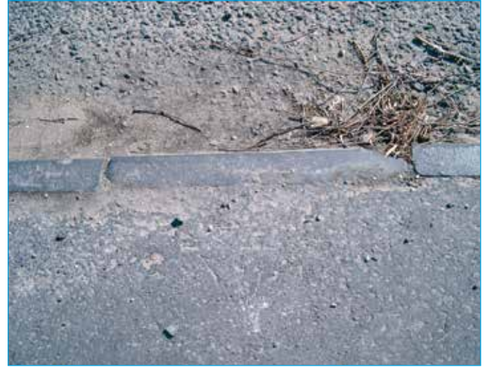
Historic blue brick kerbing and drainage, Woodhall Spa, in a Conservation Area. These should be retained wherever possible, and where replacements are necessary, these should be sympathetic. Care should be taken when resurfacing the road that this type of feature is not damaged or covered up.
