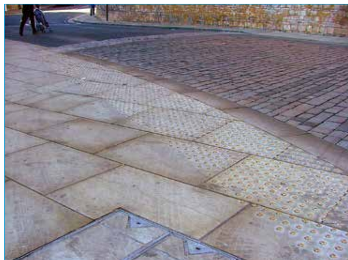
Brass studs have been used at this crossing point in Red Lion Square in Stamford. Note that the tactile paving does not need to be at right angles to the flow of traffic: they are to direct pedestrians in the right direction to meet the crossing point on the other side of the road.
