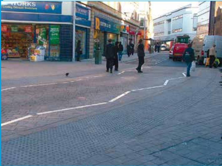
Pedestrians safely crossing Silver Street, in Lincoln's Cultural Quarter. Silver Street is a one way street, which allows for safe crossing just along from a controlled crossing without the need for guard railing. Note the continuation of the same surfacing materials from the pedestrianised areas across the crossing, but using slightly different sizes of setts laid in a different pattern to highlight the crossing area. The tactile paving is also using matching surfacing material.
