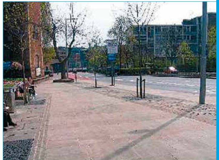
Maid Marian Way, Nottingham. Note the use of surfacing using different textures to denote areas of street furniture and trees.
