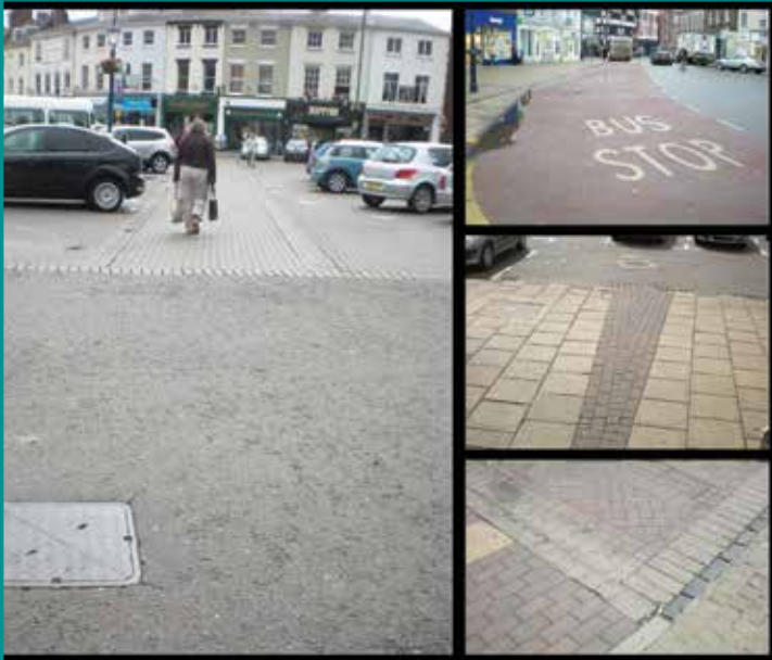
Typical materials prior to the scheme
