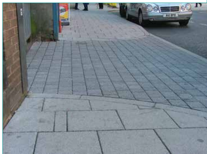
Paving on Silver Street
