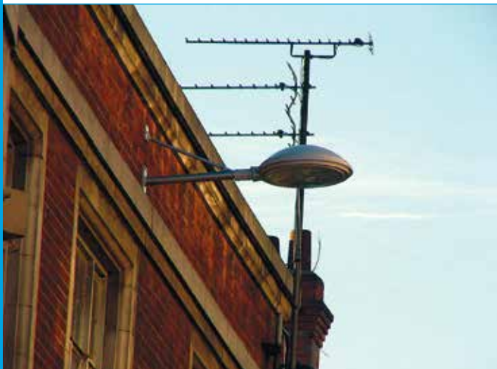
Wall-mounted street lighting equipment on a building on Clasketgate, in Lincoln's Cultural Quarter. This is a contemporary design in a Conservation Area.
