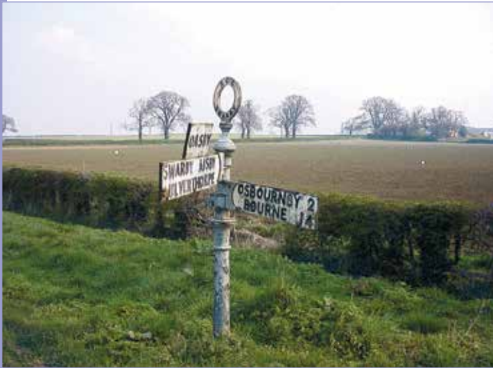
This is an example of a traditional road sign with a cast iron post and wooden arms near Swarby, before and after refurbishment. There are several variations of the cast iron posts, and these are more commonly found in the south of Lincolnshire.
