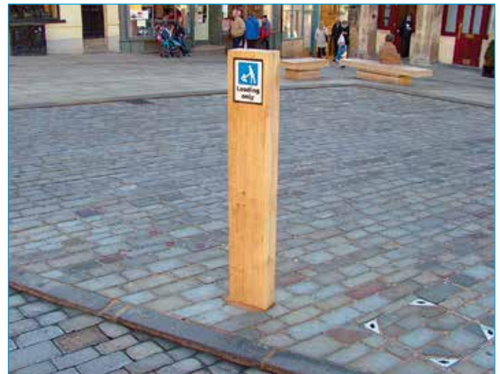
Minimal signing in Red Lion Square, Stamford. The loading bay signs are mounted on oak posts. The posts also prevent vehicles from driving onto the area adjacent to the loading bay.
