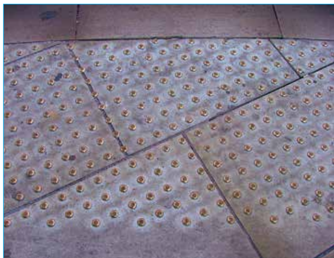
Brass studs have been used at this crossing point in Red Lion Square in Stamford. Note that the tactile paving does not need to be at right angles to the flow of traffic: they are to direct pedestrians in the right direction to meet the crossing point on the other side of the road.
