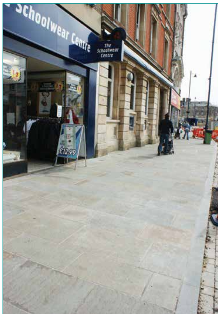
Repaved footway during construction works
