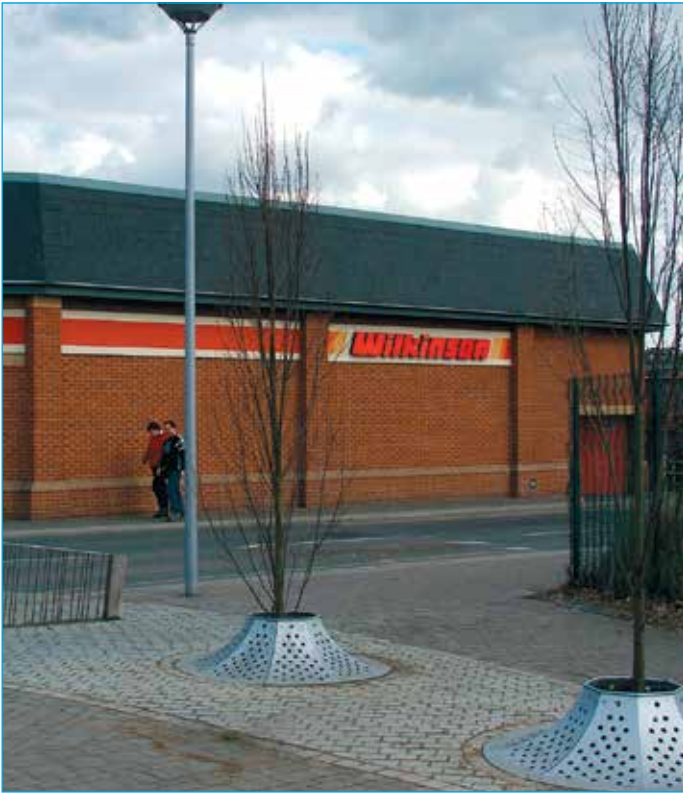
Silver Street, Gainsborough. Poorly designed tree grilles directing rainwater away from newly planted trees, these trees were replaced on a number of occasions before the grille problem was identified.
