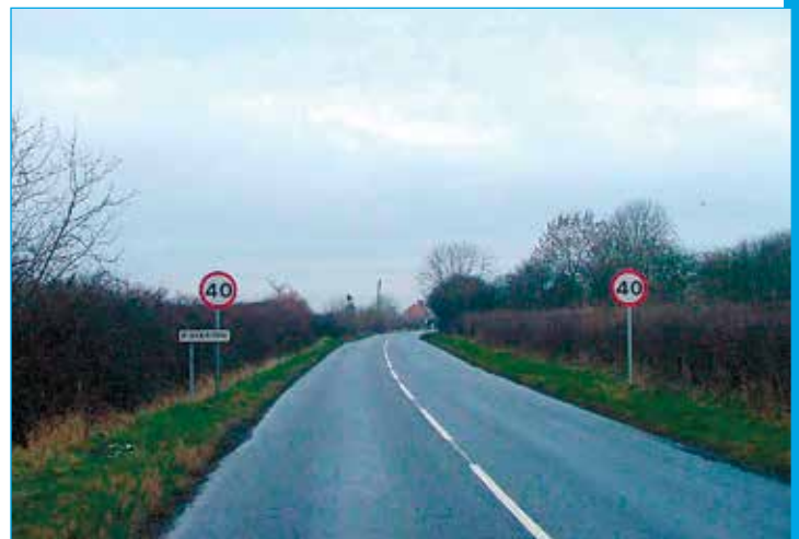
Entrance to Fiskerton with minimal signage, and no road markings.
