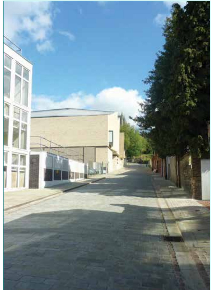
Danesgate after completion
