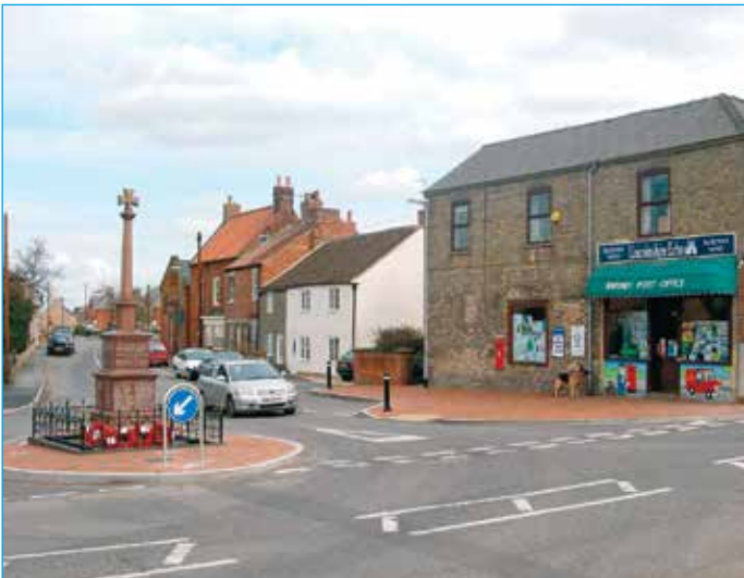
Bardney village centre improvements. Note the tightening of the junction by the installation of a build-out for pedestrians outside the Post Office.
