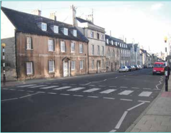
High Street St Martins before the scheme was carried out.
