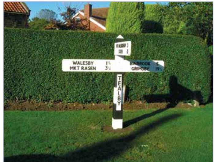
Concrete posts with wooden arms, like this example in Tealby, are more prevalent in the north of the county. Note the replacement of the modern reflective metal directional arms with wooden arms.
