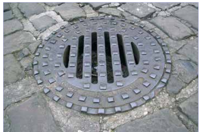
This access cover is located on Steep Hill in Lincoln, and probably dates to the first half of the twentieth century. There are other examples which survive, made by local companies, which should be retained and protected, wherever possible.
