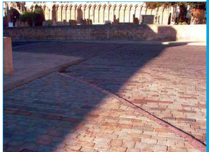
Subtle changes in surfacing materials demarcate a loading bay in Red Lion Square, Stamford. Note that there are no associated road markings.
