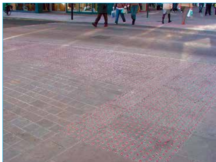
Use of distinctive design for contrasting tactile paving at the controlled crossing of High Street across Corporation Street, in Lincoln's Cultural Quarter.
