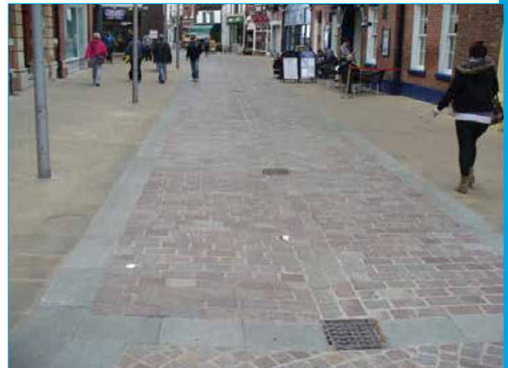
Use of level surface and complementary materials has created an attractive street scene in Lord Street, Gainsborough.
