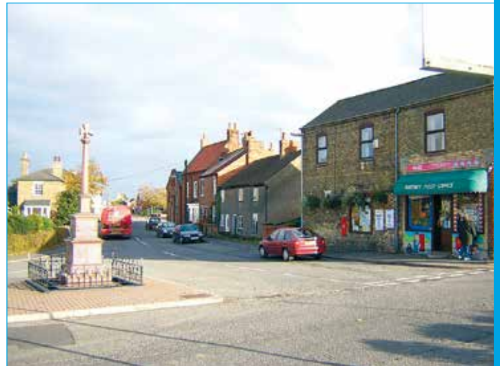
Bardney village centre improvements. Note the tightening of the junction by the installation of a build-out for pedestrians outside the Post Office.
