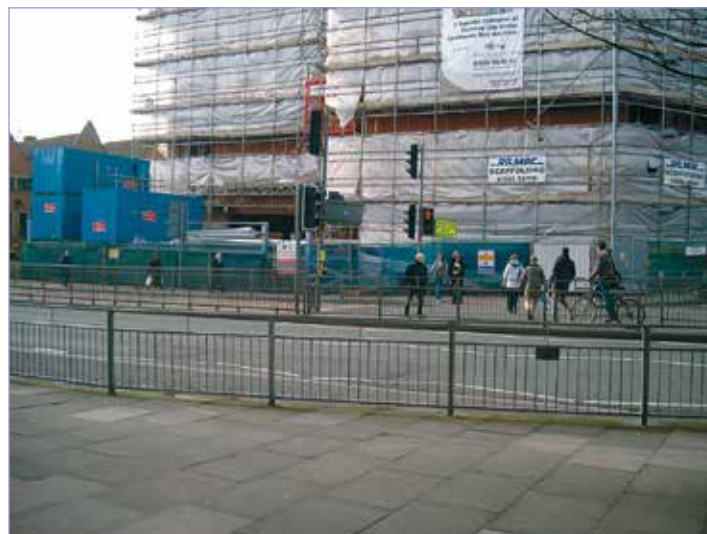
Guard rails at the pedestrian crossing on Broadgate, Lincoln. Guard rails are a potential hazard to those with Guide Dogs.
