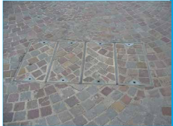
Access covers located in Gainsborough Market Place. Note the decorative pattern used to lay the setts.
