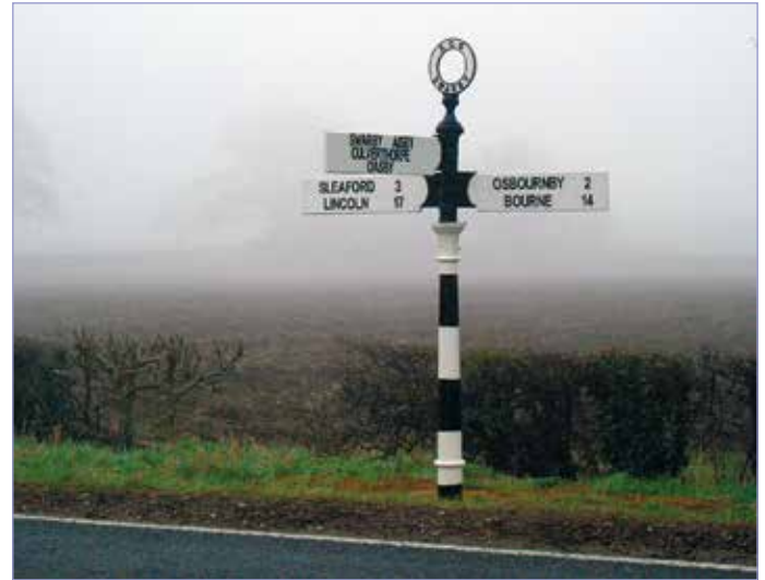
This is an example of a traditional road sign with a cast iron post and wooden arms near Swarby, before and after refurbishment. There are several variations of the cast iron posts, and these are more commonly found in the south of Lincolnshire.
