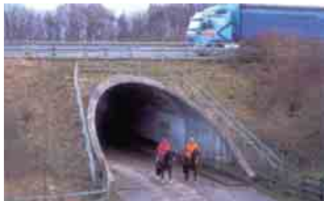
Figure 6/7 – Underpass Suitable for all NMUs
