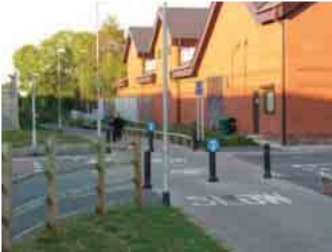
Figure 6/2 – Cycle Priority Crossing on Cycle Route at Access to Supermarket in Hereford
