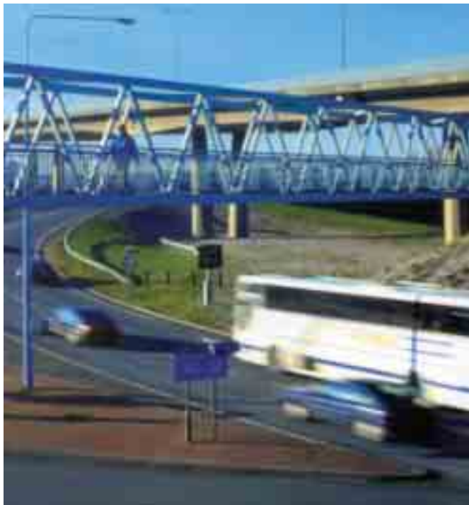
Figure 2/1 – Pedestrian Footbridge Over M1 Slip Road
