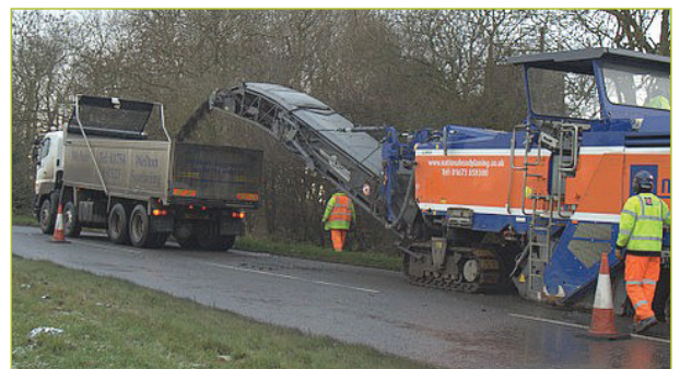
Maintenance works on the A153
