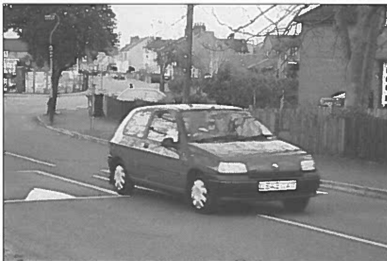
Speed cushion used in a residential area to reduce speed related accidents.
